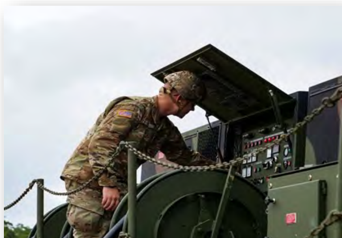
Spc. Zink parallels the generators to ensure the equipment can continue running while the previous generator is fueled.
