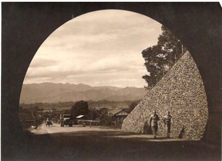
Two Soldiers walk through the tunnel on Gyoko-dori toward the main gate on what is now Highway 51. The road above the tunnel has connected south and north posts since November 1936.
