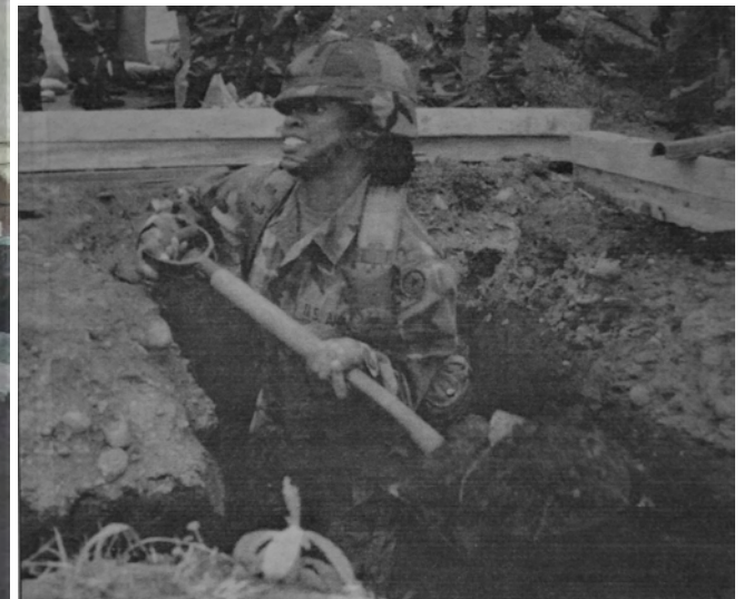
Sergeant Erika Baker digs in constructing a fighting position May 11, 2000, during a 17th Area Support Group training event at Sagami General Depot.
