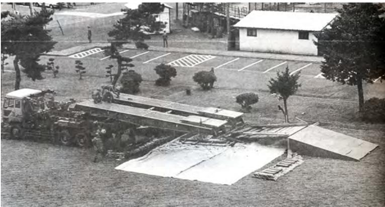
A Japan Ground Self-Defense Force crew work on placing a portable bridge over a simulated river next to a collapsed bridge. The demonstration was part of 3rd Engineer Group celebrating its 20th anniversary Oct. 11, 1992, as well as the 21st anniversary of the JGSDF subpost at Camp Zama.
