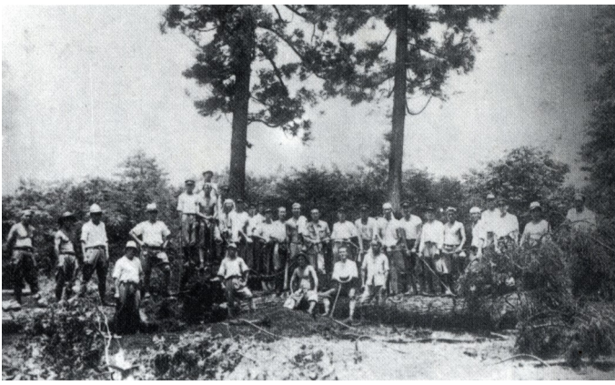
Workers take a break from building Gyoko-Doro (today's Highway 51) to pose for a photo.
