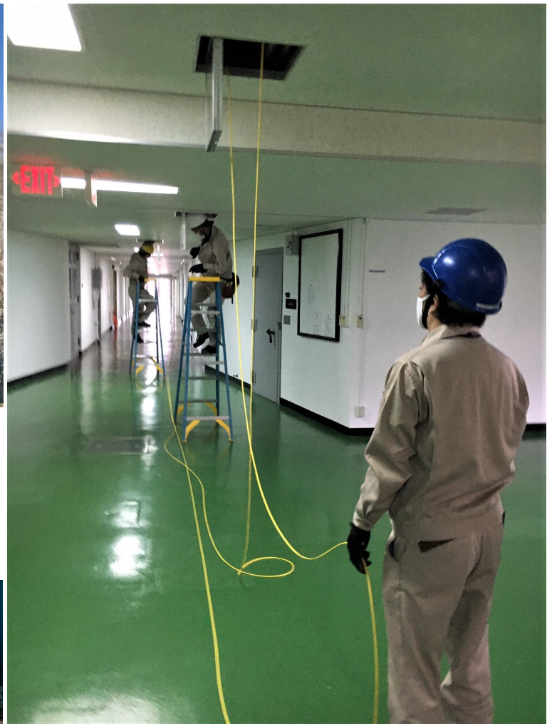
Workers from the 78th Signal Battalion's outside plant string fiber optic cable Dec. 9, 2020, for a 311th Military Intelligence Battalion project. The cable was being strung in the U.S. Army Japan headquarters building.
