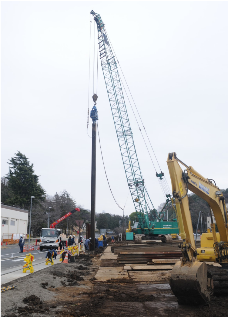
A Japanese construction crane lifts an I-beam from a section of tunnel running beneath Camp Zama on Feb. 24, 2016. The construction then was centered around the Camp Zama Community Club. The tunnel, constructed in the 1930s, has been undergoing a widening project, which started on the west side of the base and moving slowly toward the east.
