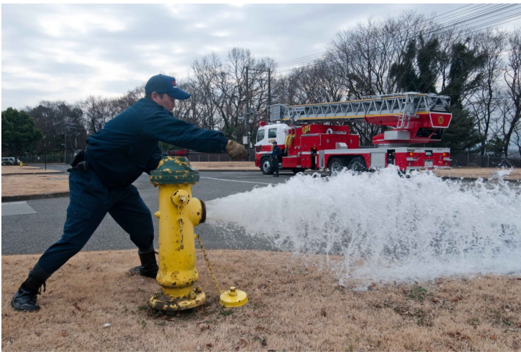
Firefighter Atsushi Komatsuzaki opens a fire hydrant valve as part of a quarterly check of Camp Zama's hydrant system in February 2013. This safety check guarantees the system is ready for emergency use.
