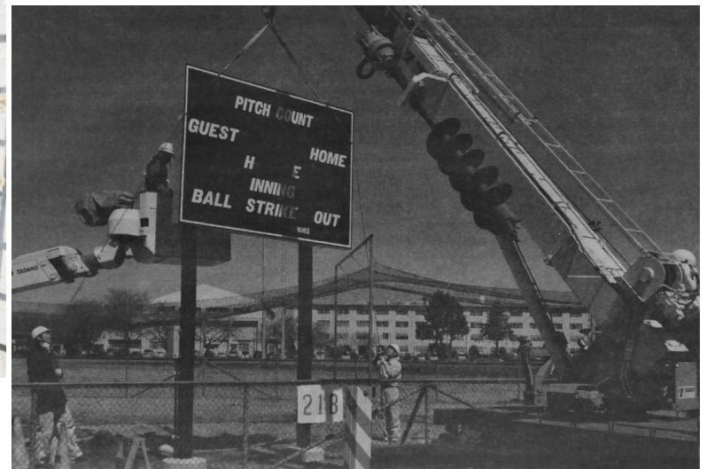
Directorate of Public Works employees install a new 70-square-foot LED electronic scoreboard April 4, 2011, at the Camp Zama softball field.
