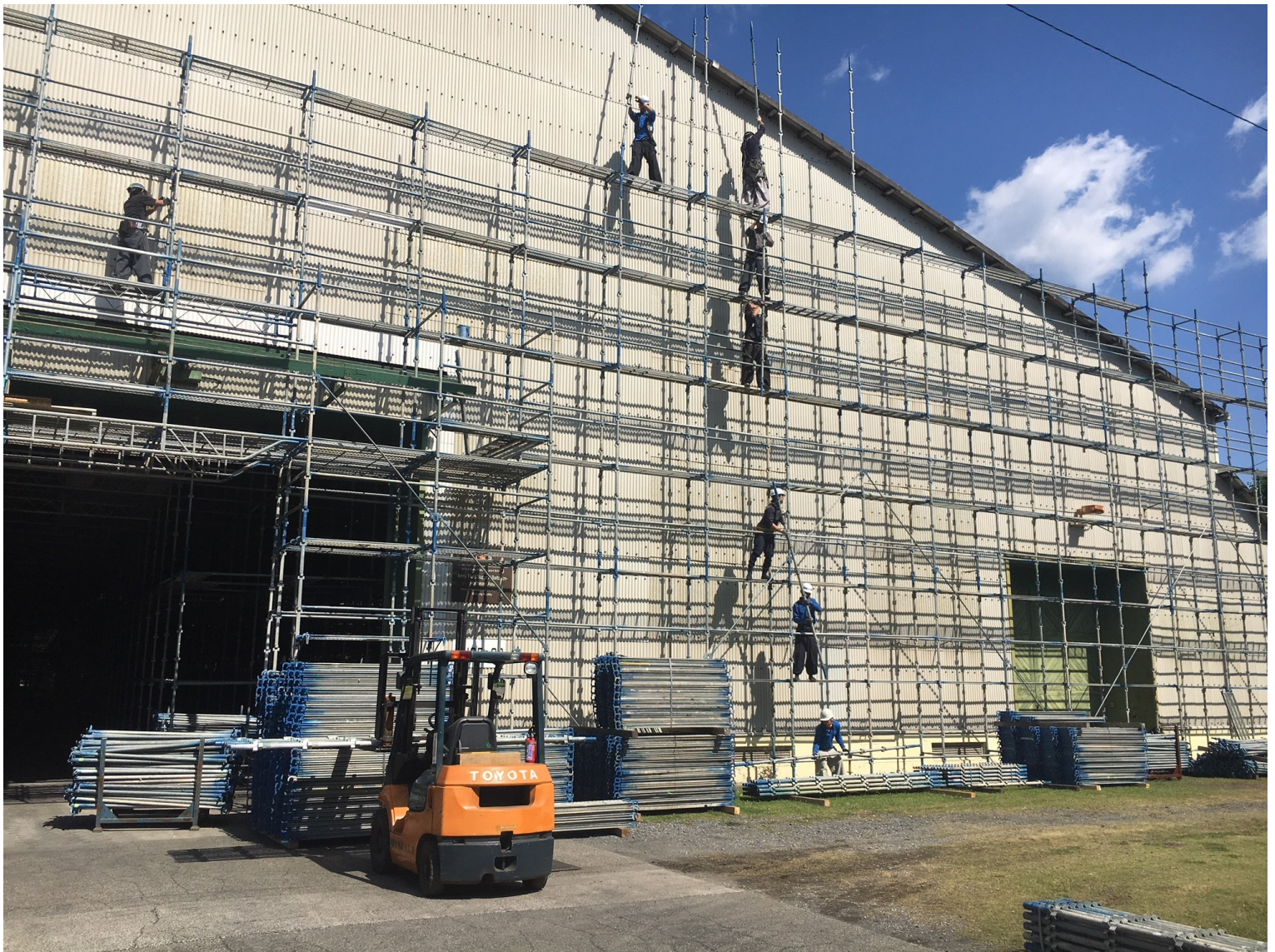
Like worker bees working on a honeycomb, contractors pass scaffolding upward for renovation of building 122-S1 at Sagami General Depot in 2017.
