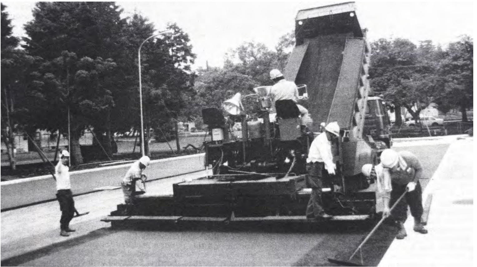
Workers pour and smooth asphalt for the new parking lot of the new Corps of Engineer District building.
