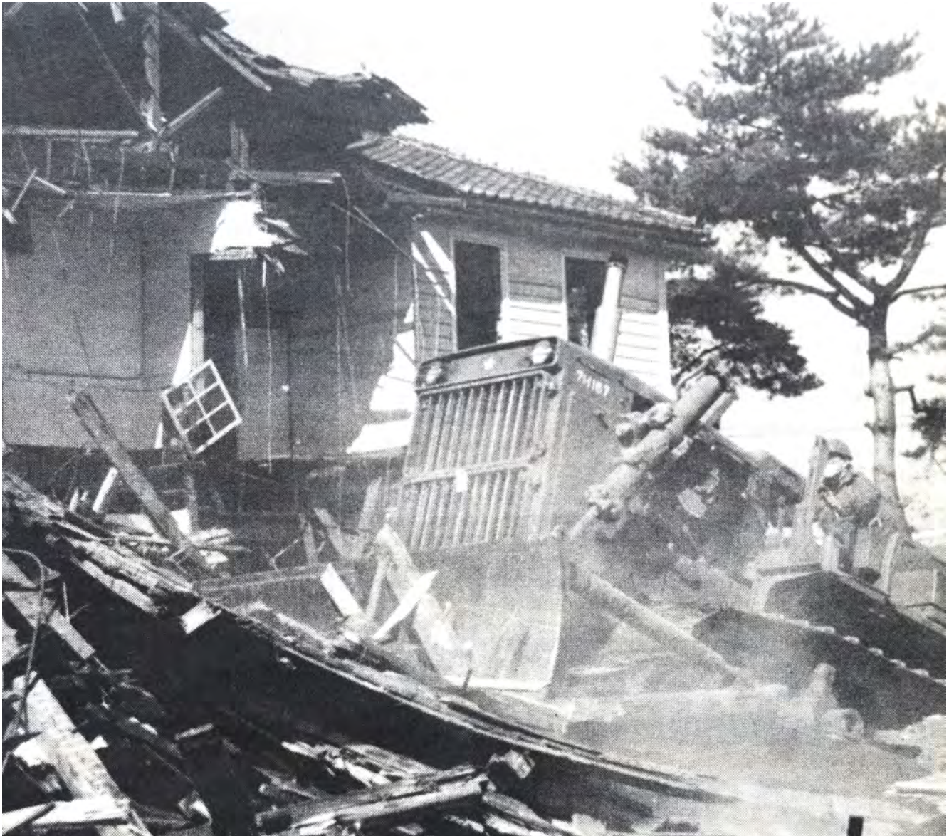
A member of Japan Ground Self-Defense Force's 3rd Engineer Group bulldozes an old building to make way for their new headquarters building on Camp Zama. JGSDF units have been collocated on Camp Zama since October 1971.
