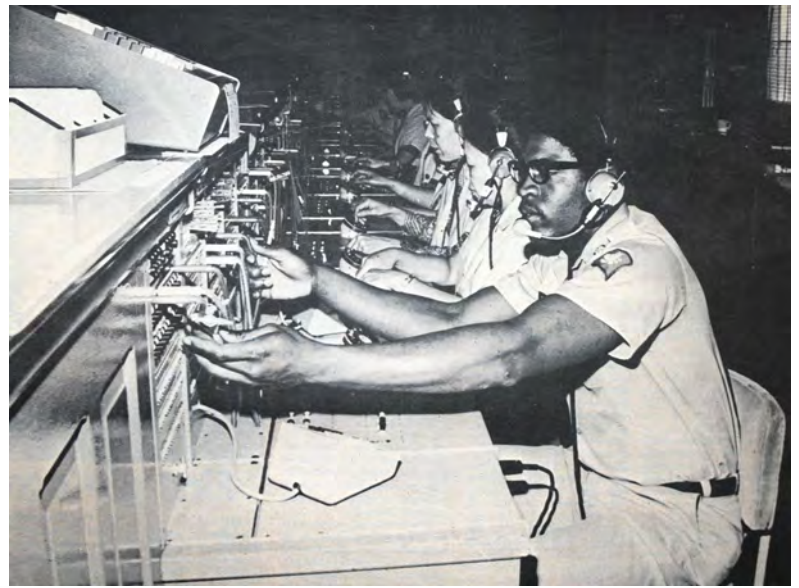
A row of telephone operators handle the switchboard
